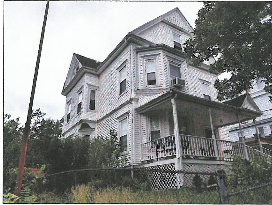
VIEW OF 40 HARVARD STREET - EXISTING CONDITION
